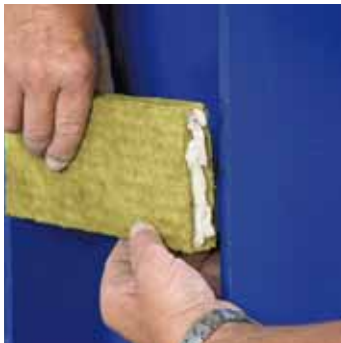
2 Pose des supports
